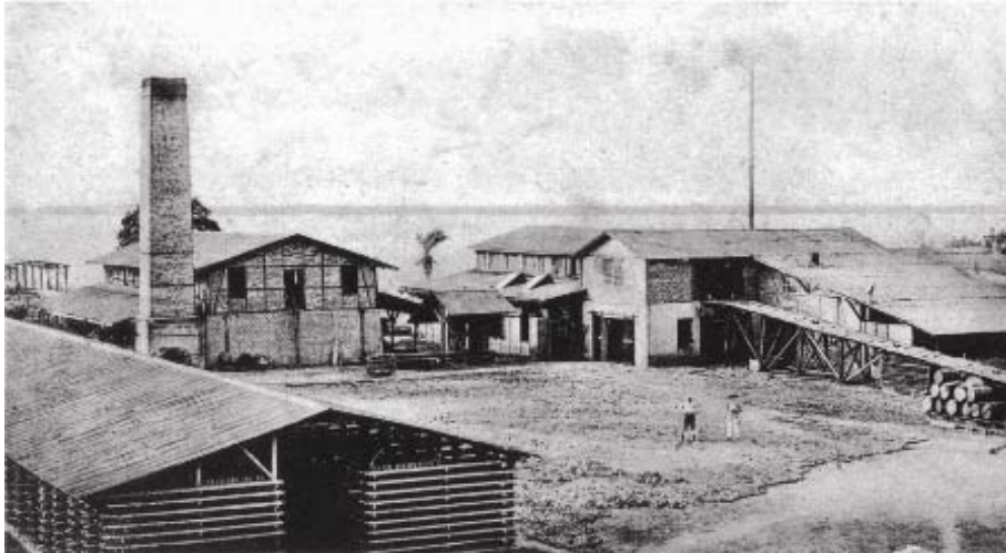
Figure 4 : German Water treatment complex [10].
