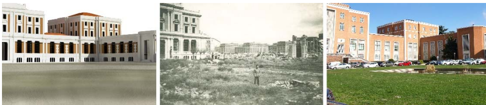
Figure 1: School of Agriculture Engineering in 1930-1939-2015. Drawing: J. Muñoz. Old photography: ETSIAAB. UPM . Current photography: J. L. González.
