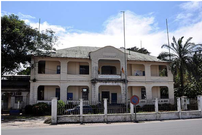
Figure 6 : Government Headquarters in Douala [12].
