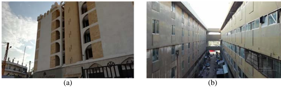
Figure 6: Industrial buildings within the site. (a) Timber factory; (b) the concrete ‘giant’.
