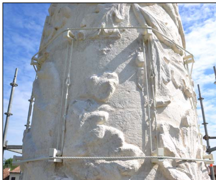
Figure 9: Stainless steel cables used to strengthening in flexure the shaft.
