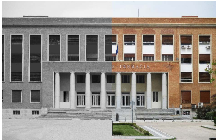
Figure 5: Façade of the Faculty of Pharmacy in 1936 and 2018 (J. L. González).
