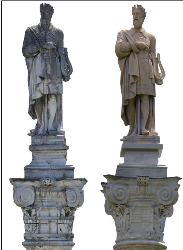
Figure 11: the capital, the podium and the statue before (left) of the restoration work and after (right).
