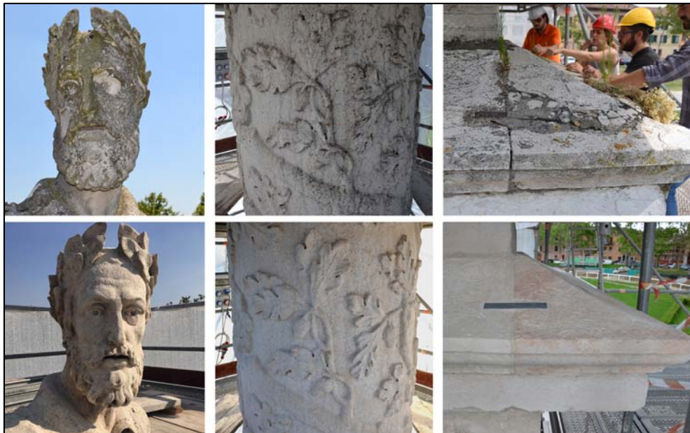
Figure 10: Operations to clean the surfaces of the statue, shaft and pedestal.
