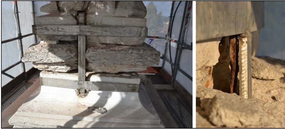
Figure 4: Podium of the statue. The external metal support ring in stainless steel has been welded to the damaged parts, accelerating oxidation.
