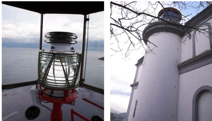
Figure 8: Acrylic optics of 2008 on white-coloured base placed on the optics implemented in 1943, with inclined struts (both work with flashes of the lamp with no rotation mechanism). Detail of the semi-embedded tower in the living quarters, office and store building.
