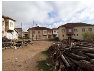
Figure 9: Buildings entered from the street
