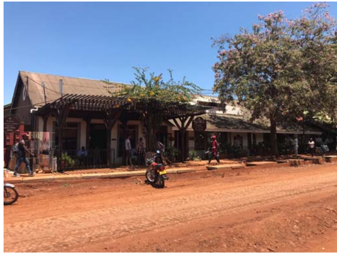
Figure 8: The Source café building 2018 [Jim Joel Nyakana]
