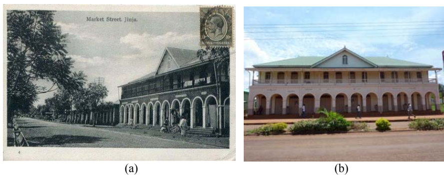
Figure 7: Madhvani Building: (a) in 1920s [36] and (b) in 2016 [author]
